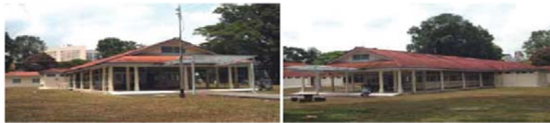
Figure H.1 Two views of the single-storey tuberculosis inpatient ward; the perimeters are free from obstruction, allowing natural ventilation throughout the year
